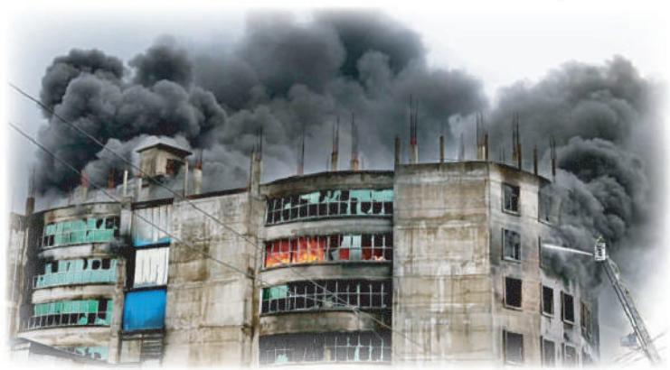
six-story juice factory in Narayanganj
